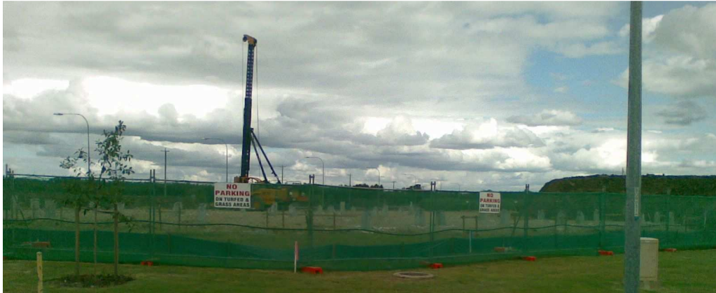
Figure 2 - Piling and foundation work as at May 09
